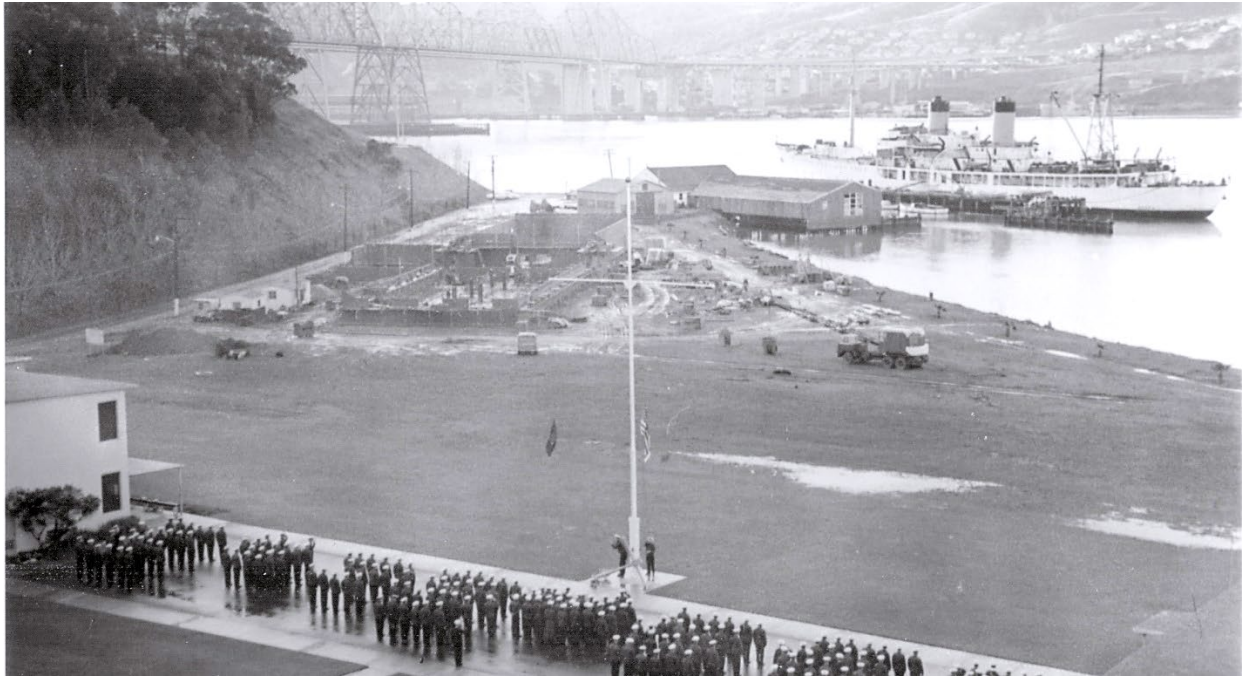
Figure 45: View of the campus looking south, c. 1959, with foundations underway for Dwyer Hall. East façade of Boathouse is visible in background. Source: Cal Maritime Campus History Collection.
