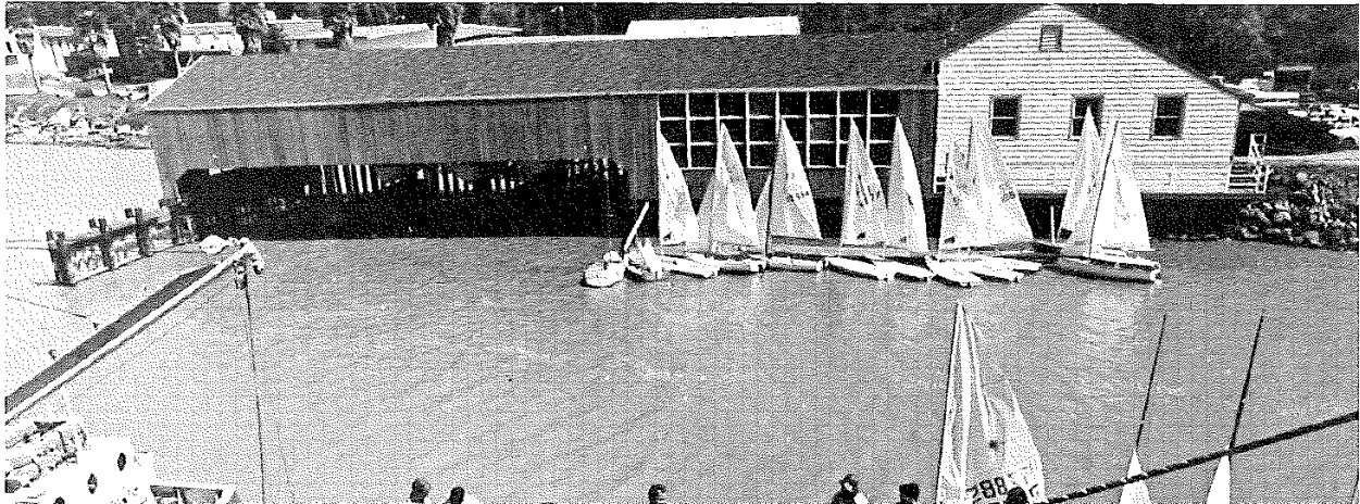
Figure 49: West façade of the Boathouse, c. 1978. Source: Hawsepipe , 1978, Cal Maritime Campus History Collection.
