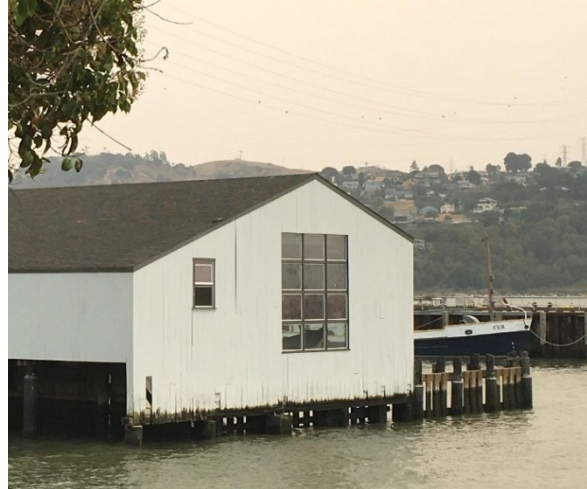
Figure 10: North façade of Boathouse, looking southwest.
