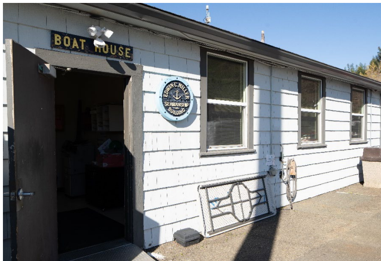
Figure 4: Detail of east portion of the south façade. Looking northeast.
