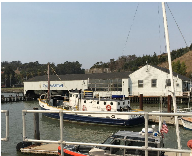
Figure 11: West façade of the Boathouse as seen from the Cal Maritime dock, looking east.
