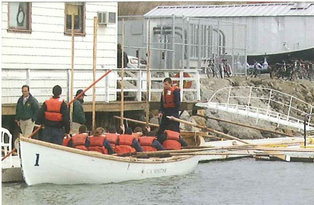
Figure 38: View showing the west façade of the Sail Loft portion of the Boathouse, 2008. Source: Hawsepape , 2008, Cal Maritime, Campus History Collection.
