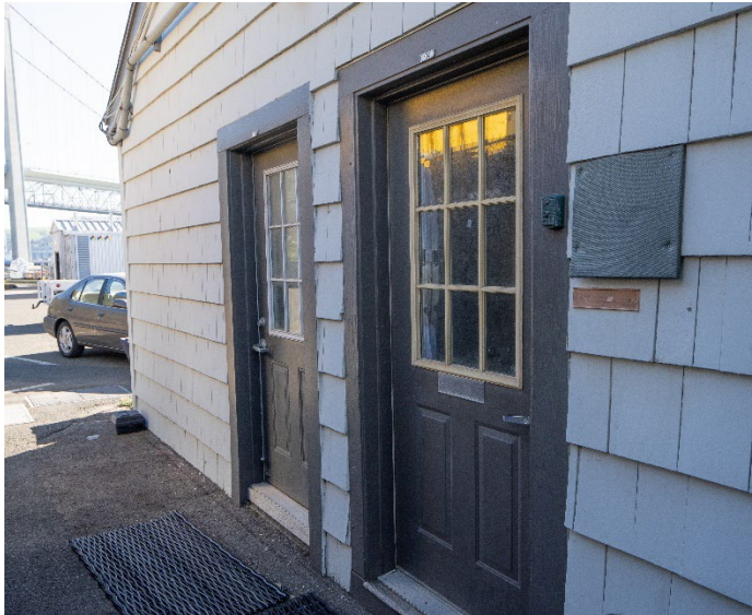
Figure 5: Detail of doors at east façade of the sail loft portion of Boathouse, looking south.
