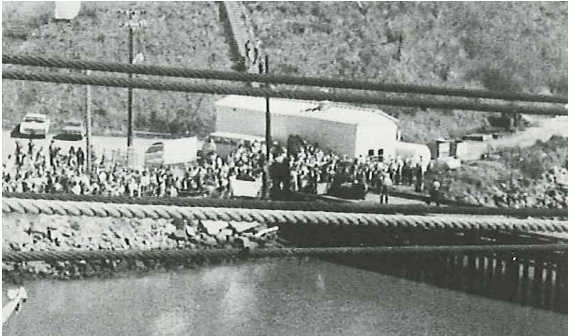
Figure 16: View east from the training ship to shore, showing south and west facades of subject building, 1978. Source: Hawsepipe , 1978, Cal Maritime Campus History Collection.
