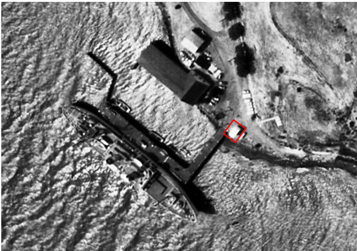
Figure 11: Aerial view of the southeast end of the Cal Maritime campus, 1965. Subject building indicated with red outline. Source: Cartwright Aerial Surveys, Flight 65-130, Frame 50-148, 1965. Courtesy of UCSB Library Geospatial Collection. Edited by Page & Turnbull.
