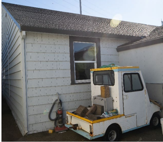
Figure 9: North-facing wall of sail loft portion of Boathouse. Looking slightly southwest.
