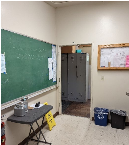
Figure 14: Looking slightly northwest from within the sail loft portion of the Boathouse.
