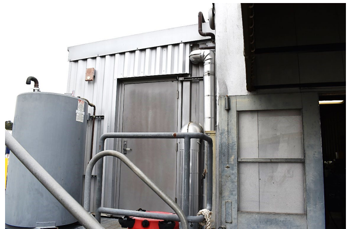
Figure 7: West end of the south facade, view northwest.
