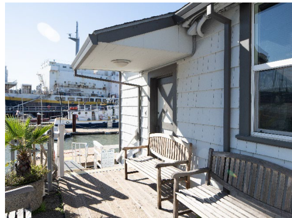
Figure 4: Detail of original primary entrance to the Boathouse, looking slightly northwest.
