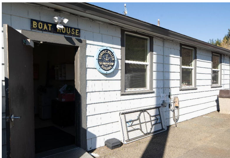
Figure 4: Detail of east portion of the south façade. Looking northeast.
