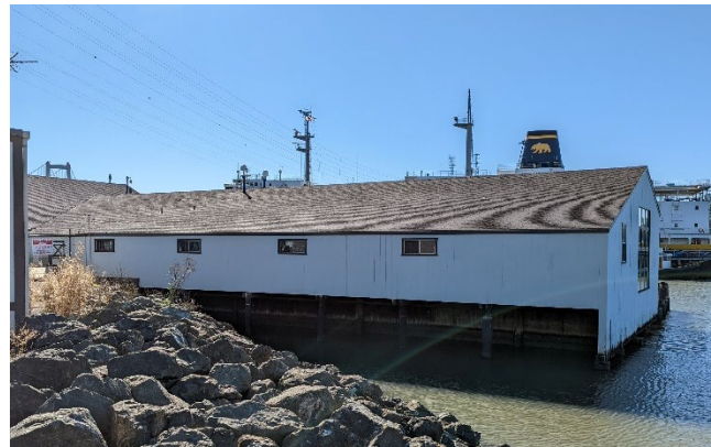
Figure 8: East façade of the transverse wing of the Boathouse. Looking slightly southwest.
