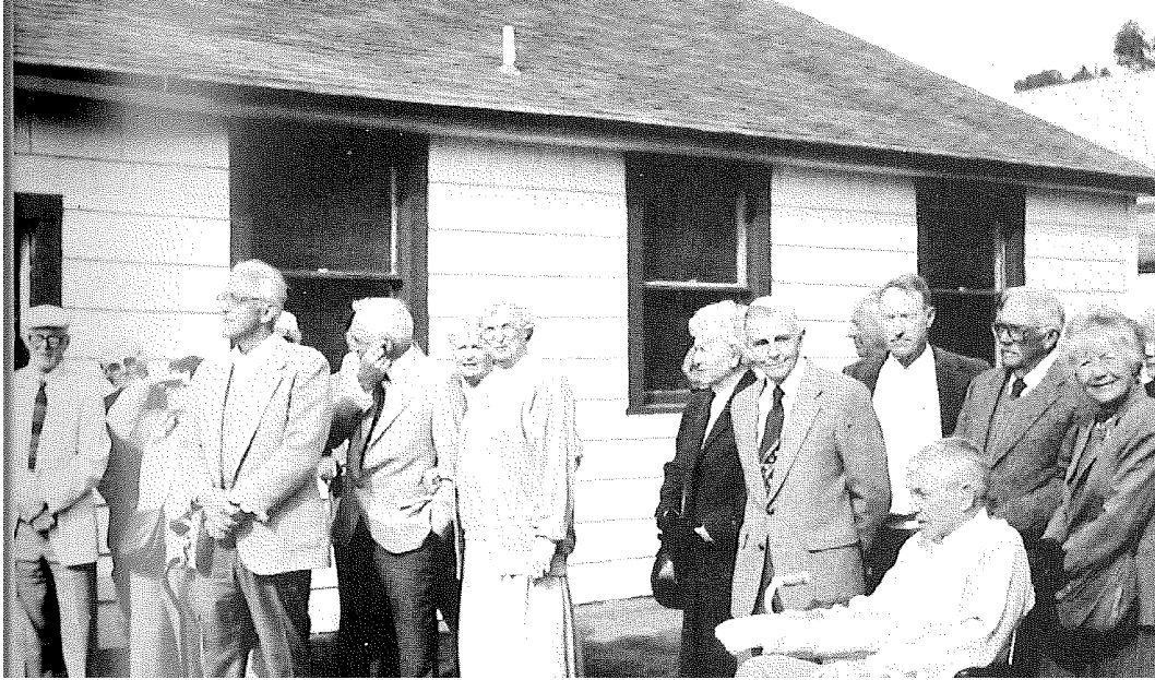
Figure 37: South façade of the Boathouse, door at far left of frame present by 1989. Source: Hawsepape , 1990, Cal Maritime, Campus History Collection.
