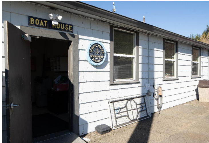
Figure 5: Detail of east portion of the south façade. Looking northeast.
