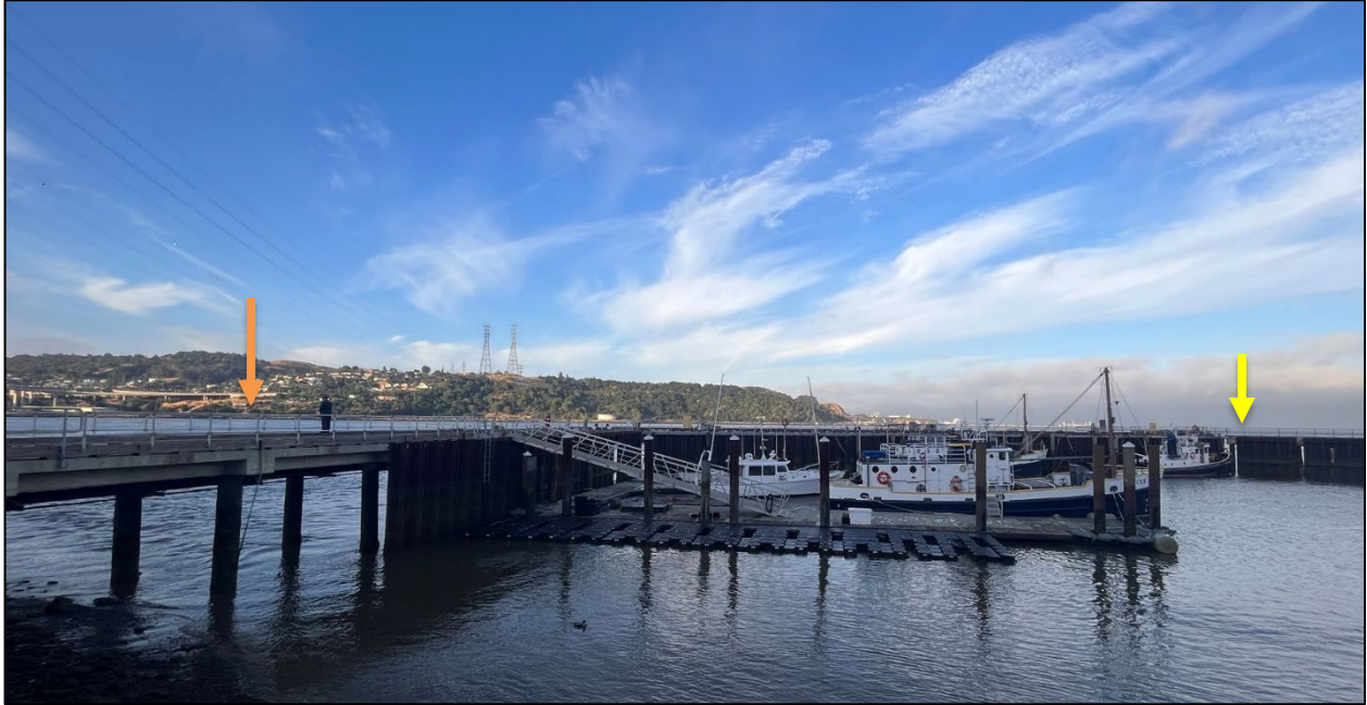
Photo 3. Looking roughly southward from the shoreline into the existing boat basin. Boat basin is within the existing breakwater with the trestle to the left (orange arrow) and main pier in the background (yellow arrow). Boat basin is within existing maintenance dredge footprint.
