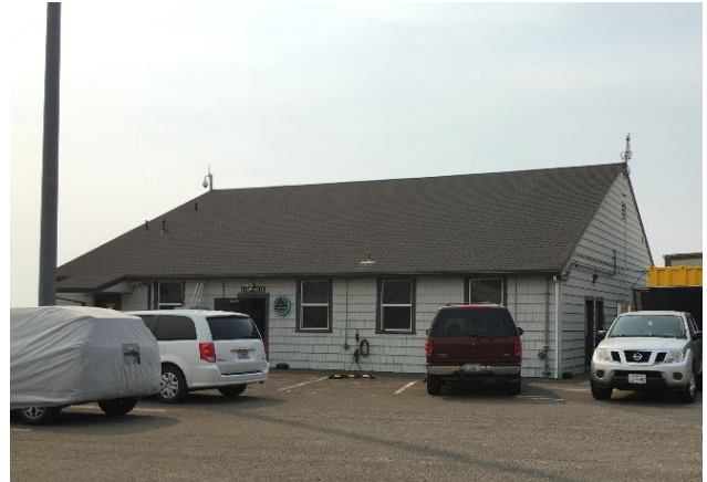
Figure 3: South façade of the Boathouse, looking northwest.
