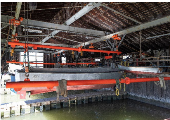
Figure 19: Looking north at the boat slips from the work platform. Note the yellow painted metal ladders from the rear storage area.
