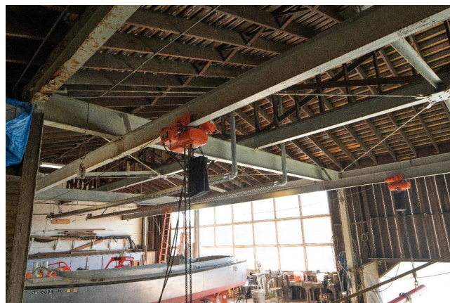
Figure 24: Looking southwest and up at metal framing of building.
