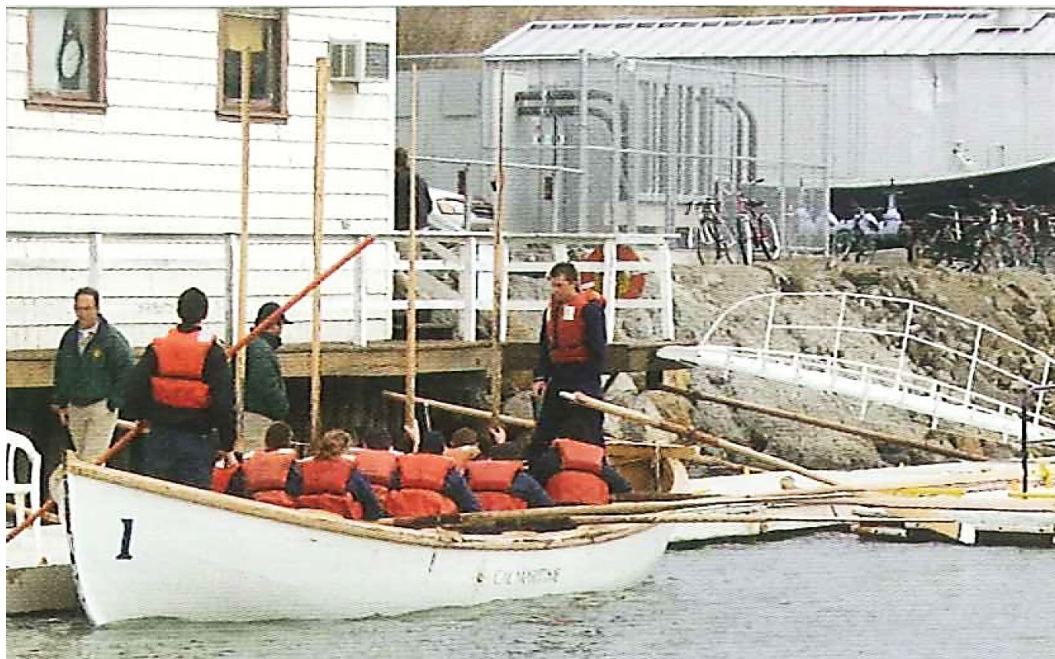
Figure 17: View showing a portion of the Boathouse's south façade (foreground) and the Machine Shop's west façade (background), 2008. Source: Hawsepipe , 2008, Cal Maritime Campus History Collection.
