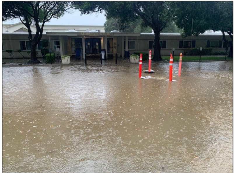
Flooding in Parking Lot A at the Administration Building (Date: 2020 1 )
