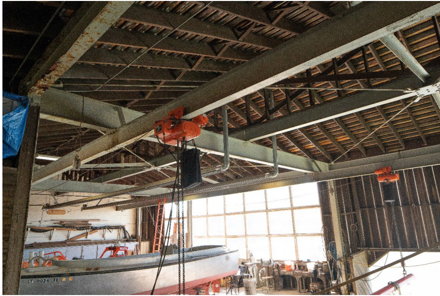
Figure 25: Looking southwest and up at metal framing of building.
