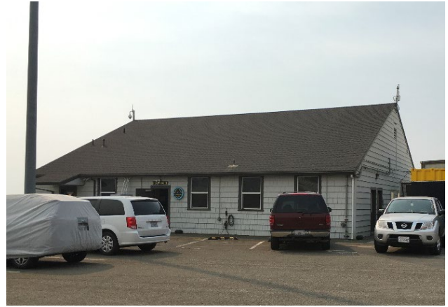
Figure 3: South façade of the Boathouse, looking northwest.
