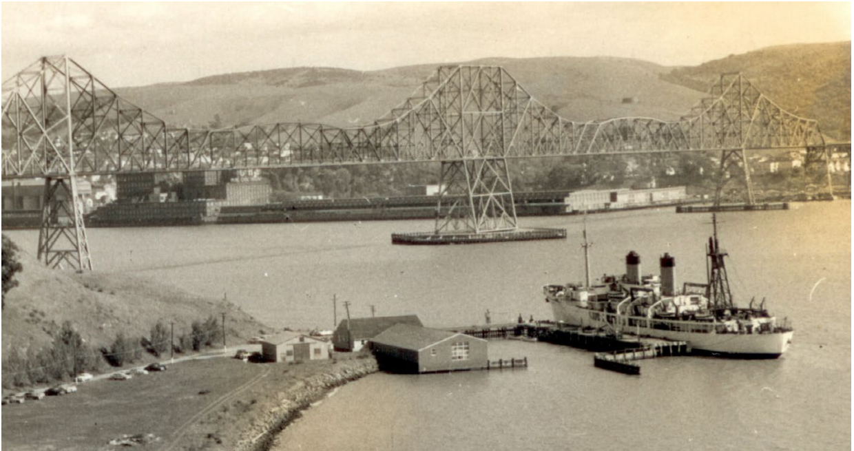
Figure 34: Looking south over the Boathouse and wharf, towards the Carquinez Bridge, c. 1948. Source: Cal Maritime, Campus History Center.
