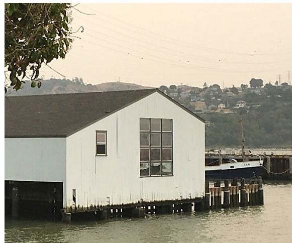
Figure 11: North façade of Boathouse, looking southwest.
