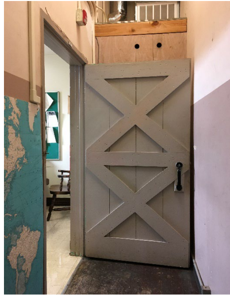
Figure 17: Original door extant in sail loft portion of Boathouse.
