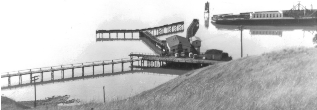
Figure 28: Photograph of Morrow Cove taken by Edwin C. Miller in December 1940, while at the site as part of a survey party of Maritime Academy administrators. Existing piers and structures were fully removed by 1946. At the far right is the Contra Costa , which served as a breakwater. Source: Cal Maritime, Campus History Collection.
