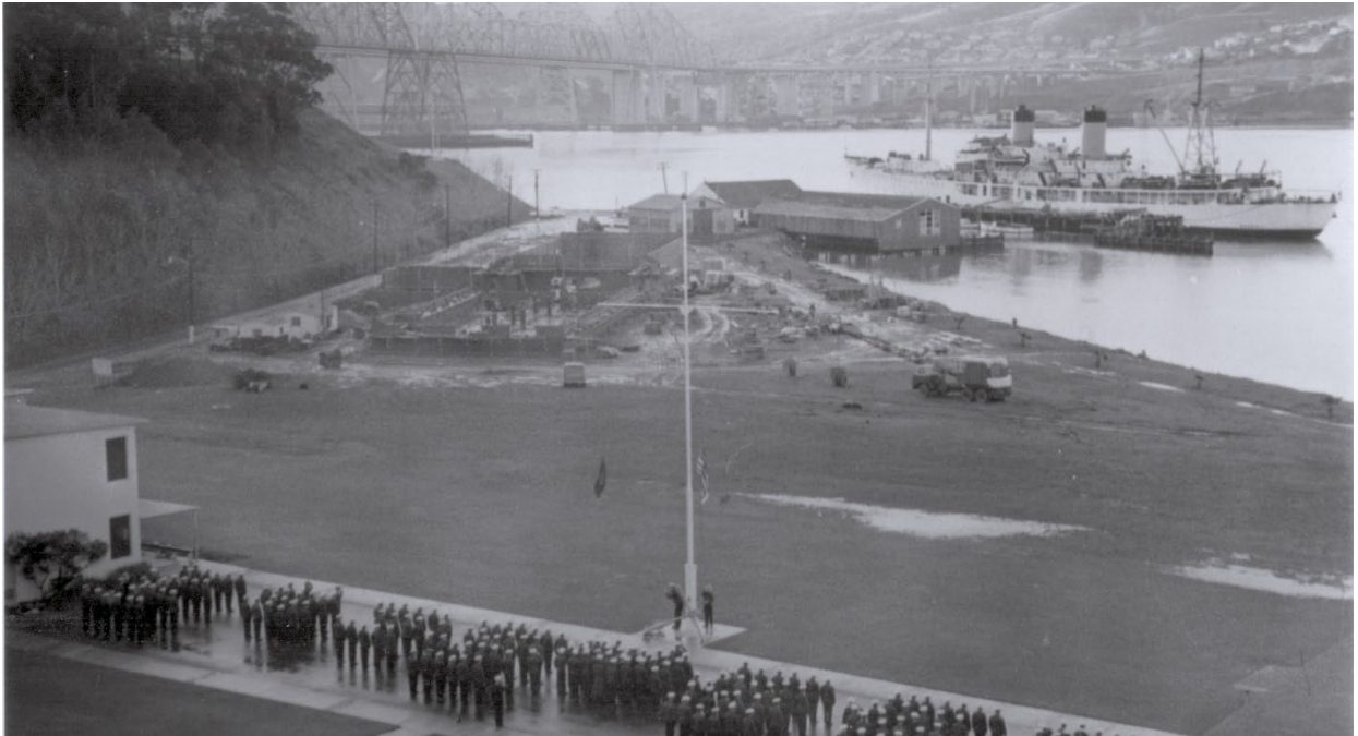
Figure 44: View of the campus looking south, c. 1959, with foundations underway for Dwyer Hall. East façade of Boathouse is visible in background. Source: Cal Maritime Campus History Collection.
