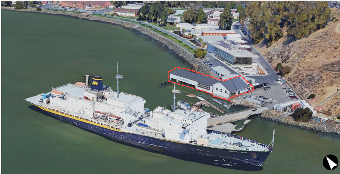
Figure 2: Boathouse at the Cal Maritime Academy campus. Building identified with dashed red line. Source: Google Maps, 2021. Edited by Page & Turnbull.
