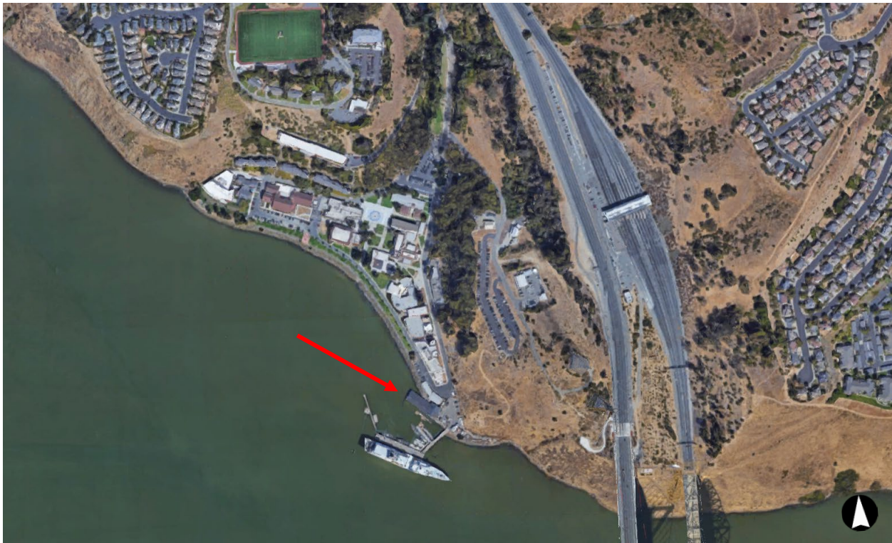
Figure 1: Aerial view of the Cal Maritime campus. The Boathouse is identified with a red arrow. Source: Google Maps, 2021. Edited by Page & Turnbull.
