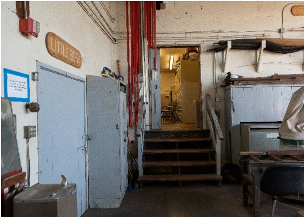
Figure 21: Looking south into the sail loft from the work platform.
