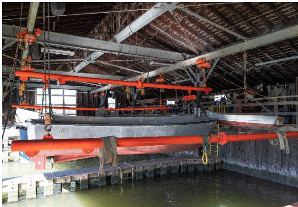
Figure 18: Looking north at the boat slips from the work platform. Note the yellow painted metal ladders from the rear storage area.
