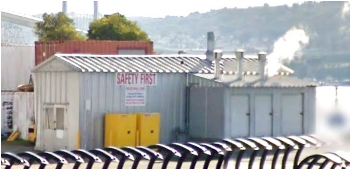
Figure 18: Oblique view of the Machine Shop's primary and west facades, view southeast, December 2016. Source: Google Street View.
