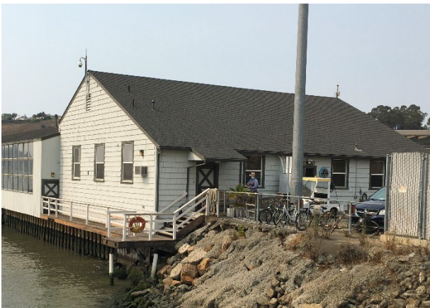
Figure 3: South façade of the Boathouse, looking northeast.
