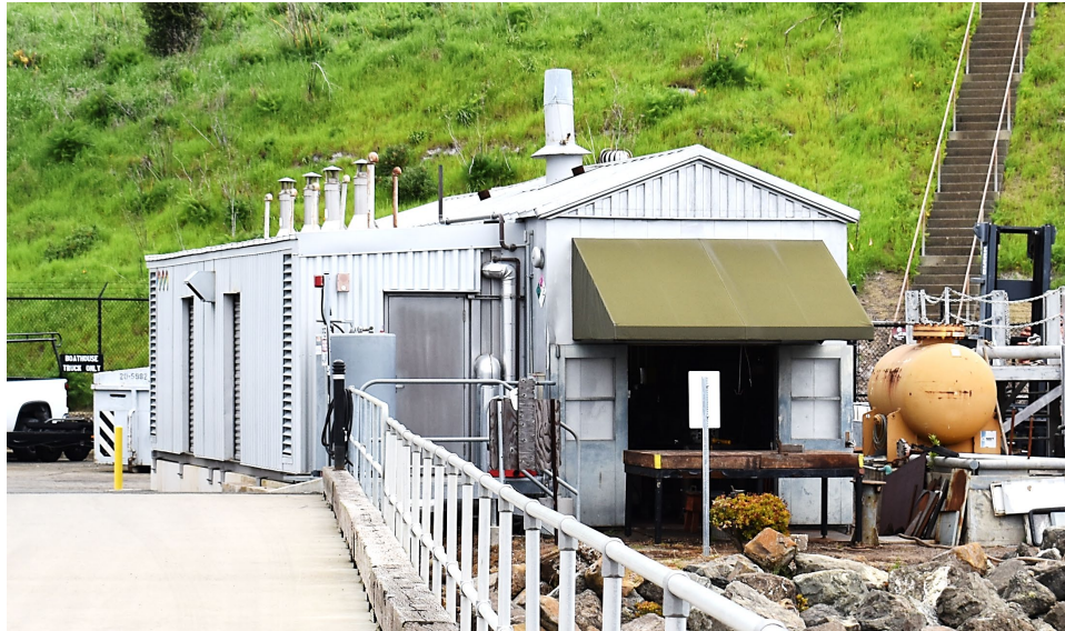
Figure 5: South facade, view northeast from pier.
