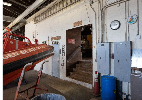
Figure 21: Looking northeast from the work platform to the elevated storage area.
