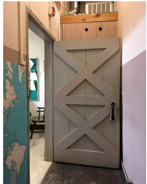
Figure 18: Original door extant in sail loft portion of Boathouse.
