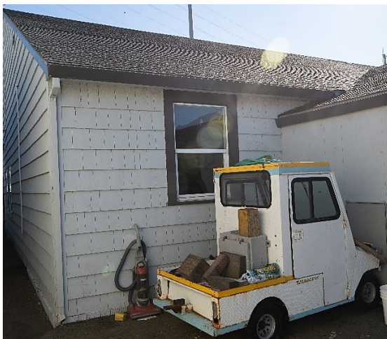
Figure 10: North-facing wall of sail loft portion of Boathouse. Looking slightly southwest.
