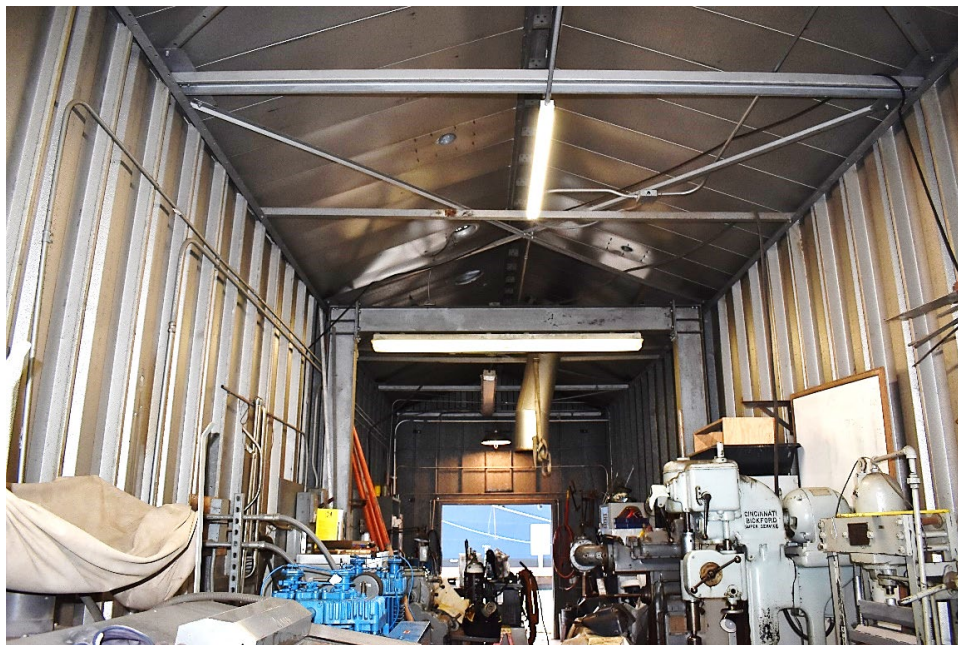
Figure 10: Interior of east volume, view northeast.
