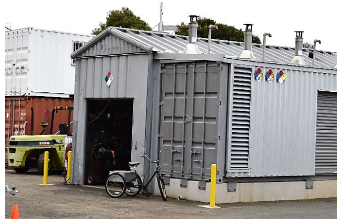
Figure 3: Oblique view of the primary facade (left) and west facade (right), view southeast.
