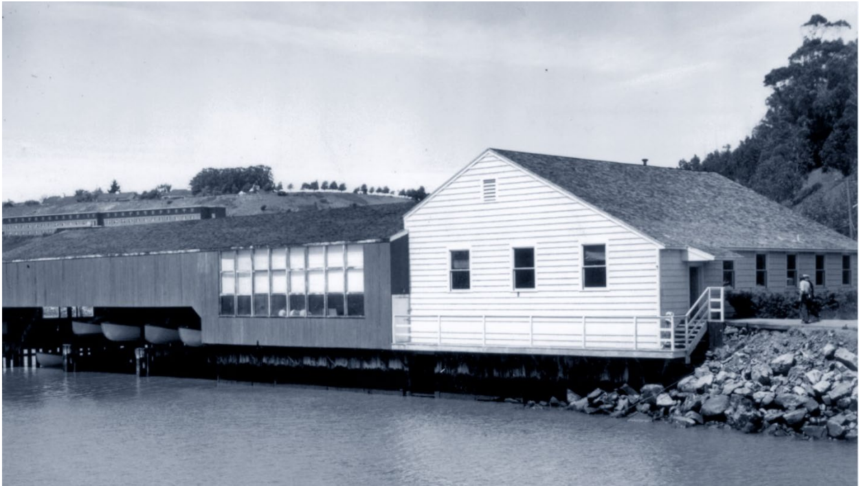
Figure 46: West and south façades of the Boathouse, 1960s. Source: Cal Maritime Campus History Collection.
