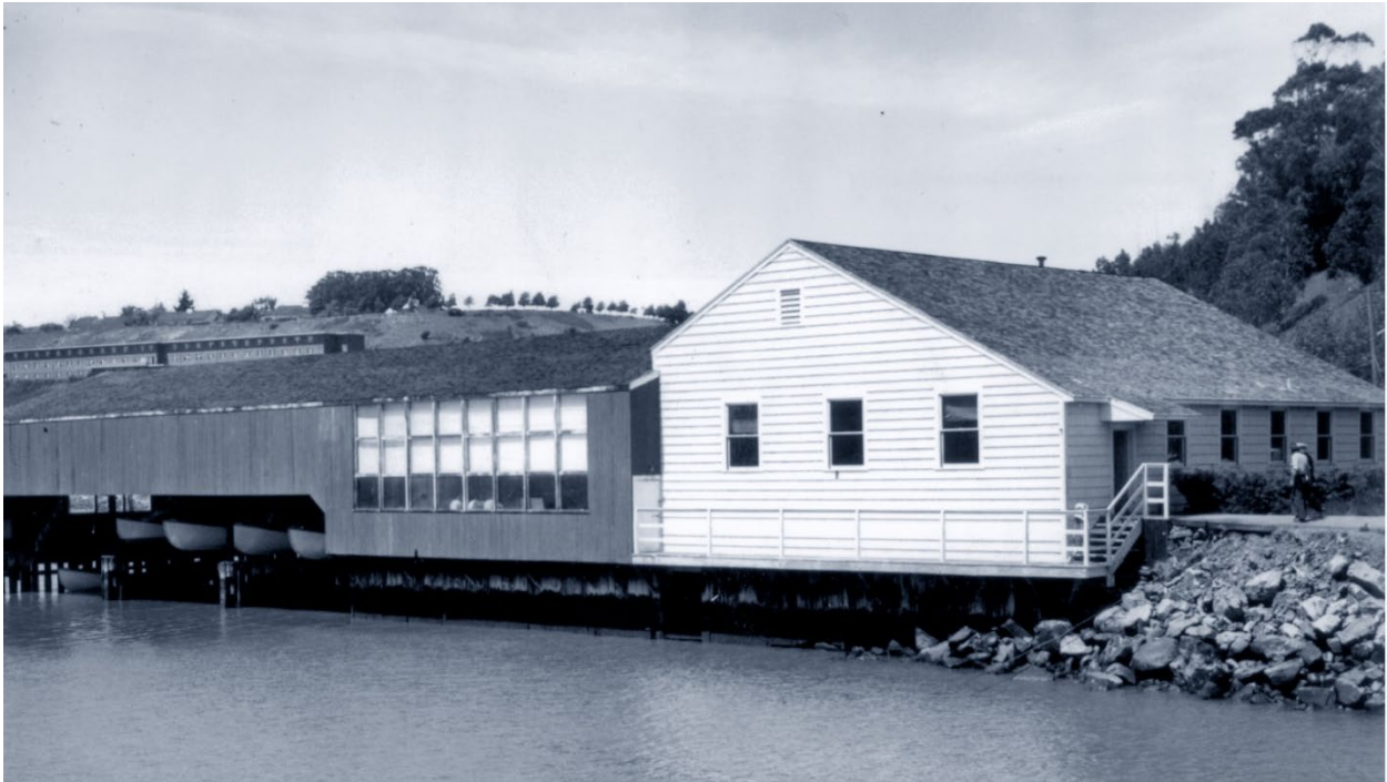
Figure 46: West and south façades of the Boathouse, 1960s. Source: Cal Maritime Campus History Collection.
