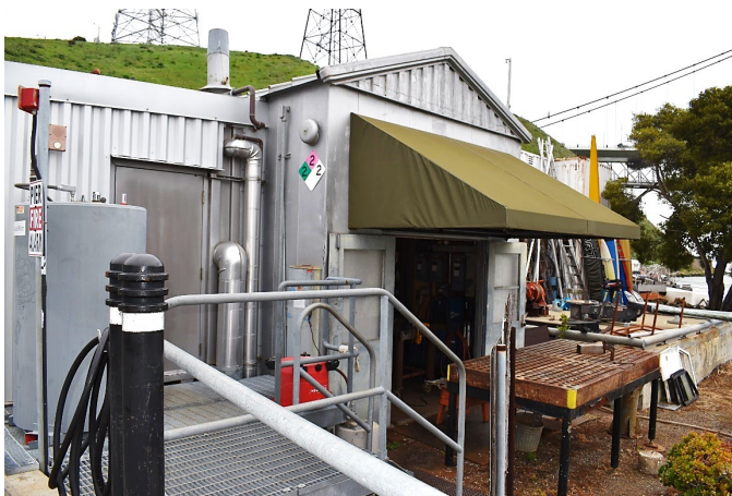
Figure 6: Awning over primary rear entrance on south facade, view east.
