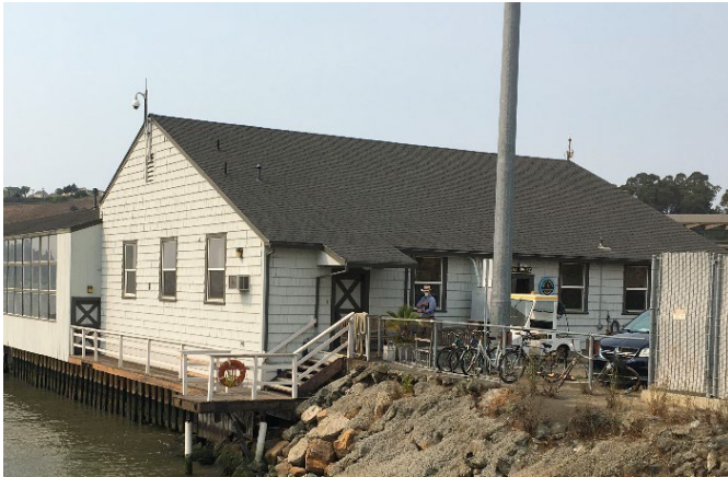
Figure 2: South façade of the Boathouse, looking northeast.
