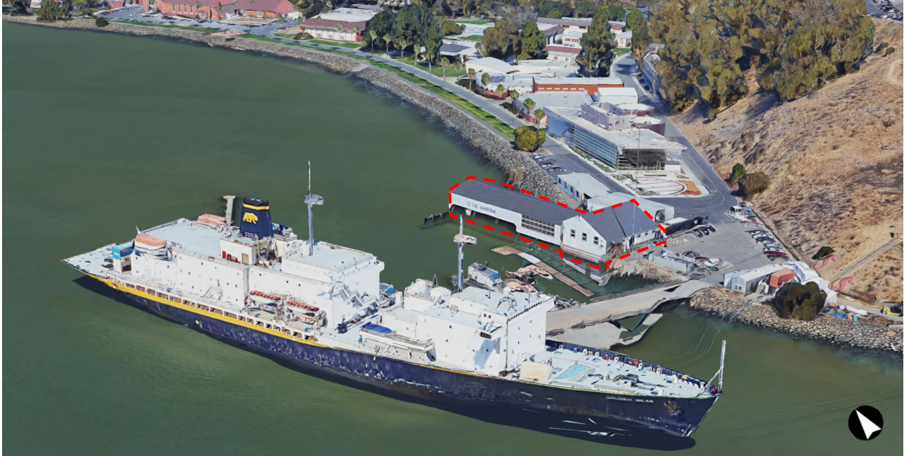
Figure 1: Boathouse at the Cal Maritime Academy campus. Building identified with dashed red line. Source: Google Maps, 2021. Edited by Page & Turnbull.
