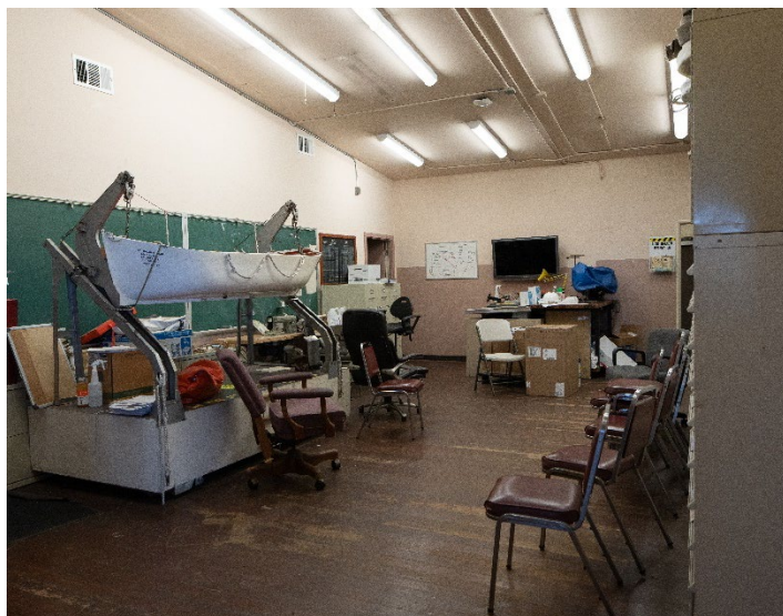
Figure 16: Original door extant in sail loft portion of Boathouse.
