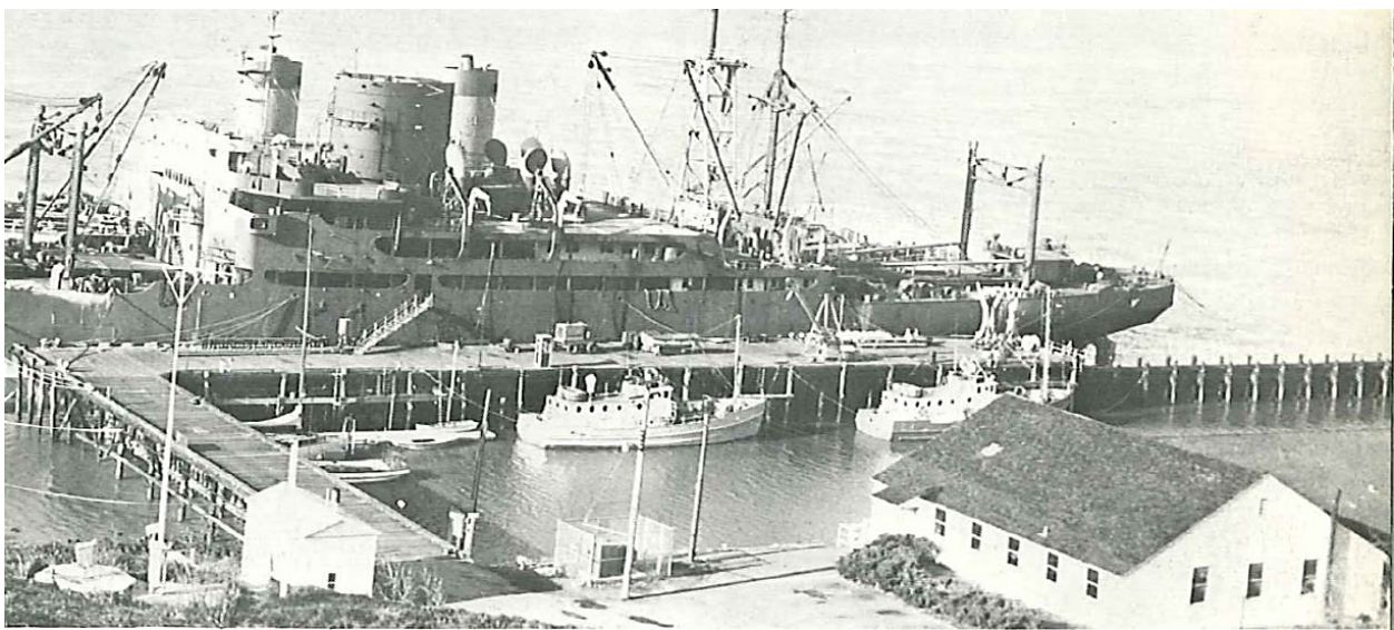
Figure 36: View of the Boathouse and wharf, c. 1971. Source: Hawsepipe , 1971, Cal Maritime Campus History Collection.
