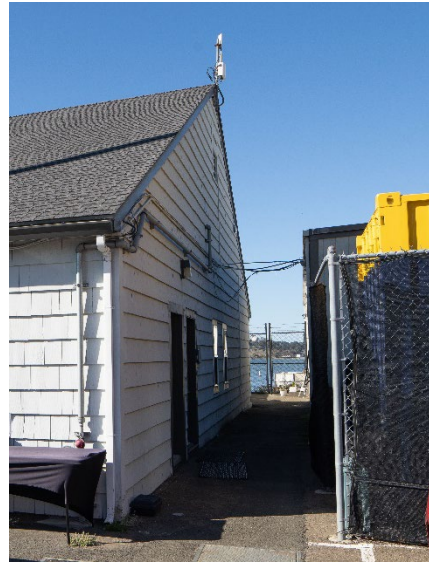
Figure 6: Oblique view of east façade of the sail loft portion of the Boathouse. Looking southwest.
