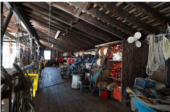
Figure 23: Looking north along the elevated rear storage area.
