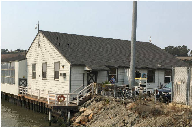
Figure 2: South façade of the Boathouse, looking northeast.
