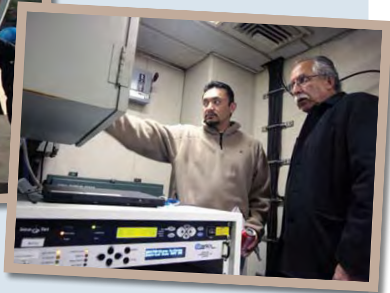
LEFT: Workers begin installing the protective fiberglass panels which surround the new shipboard satellite antenna. BELOW: Cal Maritime Network Analyst Walter Abarca shows John Rolon of the California State University Technology Infrastructure Services Department the electronic controls for the dish system.
